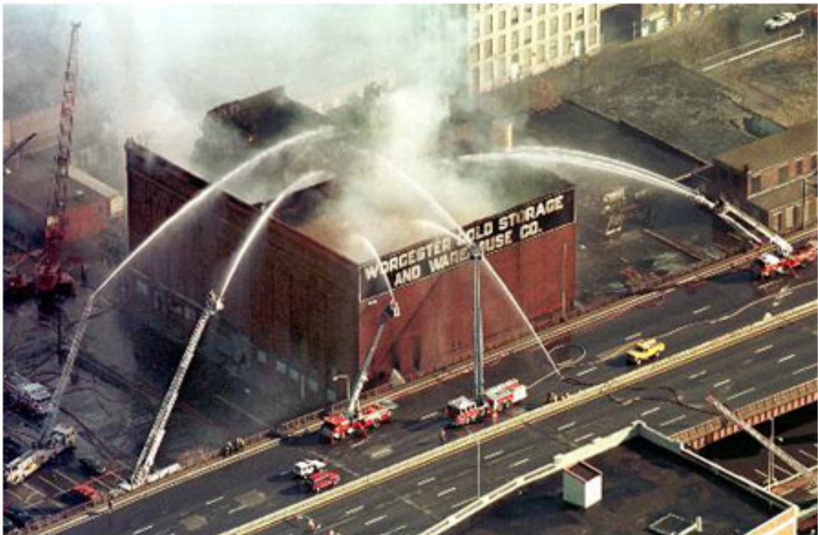
Figure 11, Worcester Warehouse Fire
